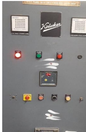
Figure 7. Tap changing transformer in powerhouse
