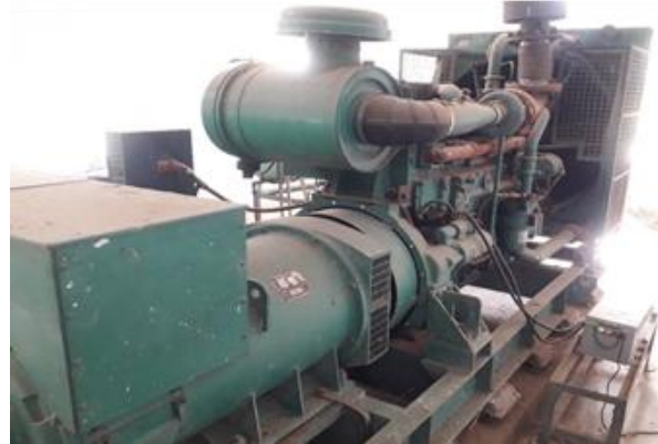
Figure 4. Diesel generator in GCT
