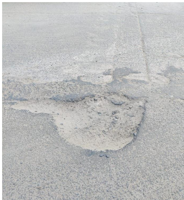
Figure 3. Detailed image of captured pothole.
