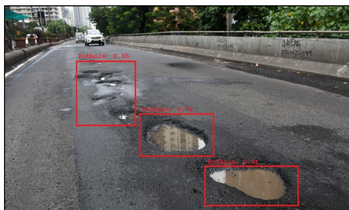
Figure 3. Pothole Detected Output
