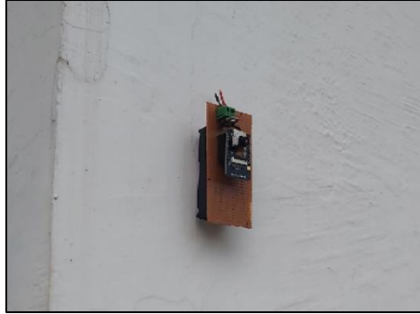
Figure 9. On-site ESP32 CAM
