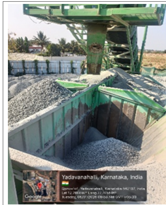
Figure 3. Aggregate storage and batching arrangement at the RMC facility
