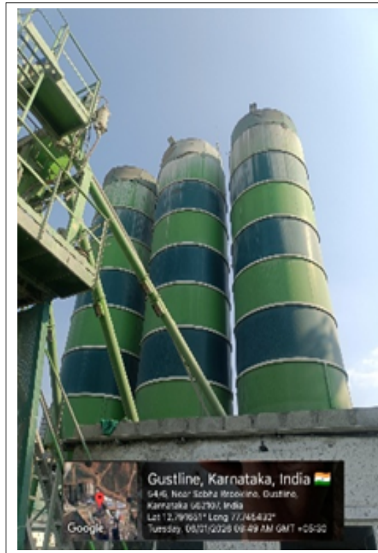
Figure 4. Cementitious-material storage silos used for RMC production
