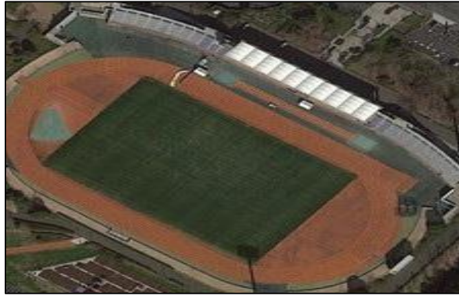
Figure 9. Failure Captioning Case
